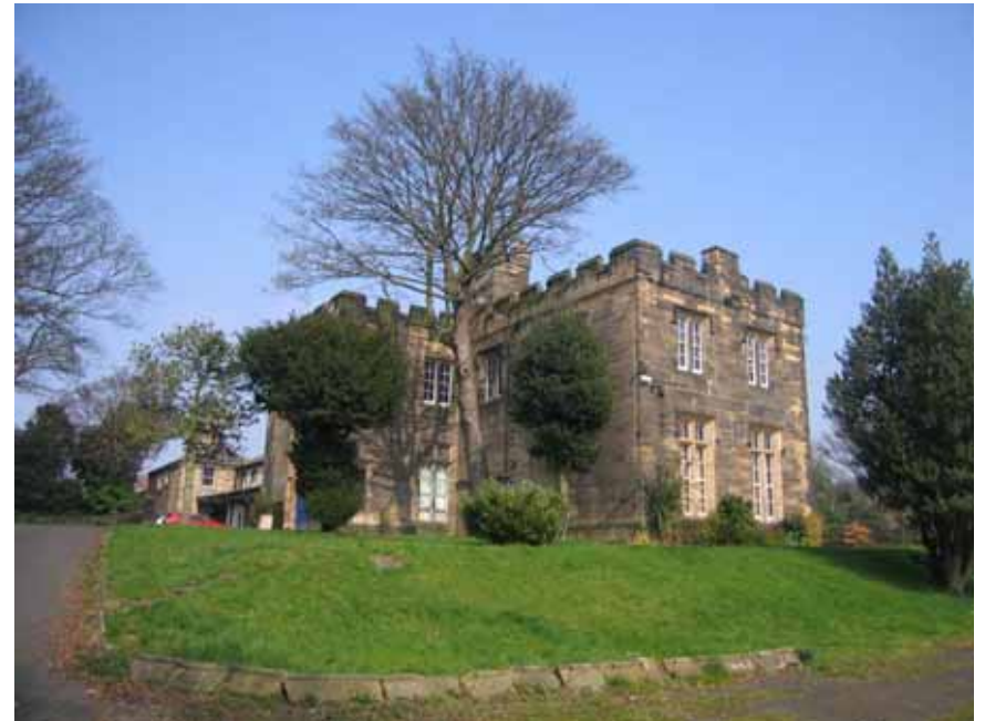
FORMER BYKER GROVE STUDIOS THE MITRE BUILDING BENWELL TERRACE NEWCASTLE UPON TYNE NE15 6LX
