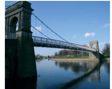
River Trent Pedestrian Bridge
